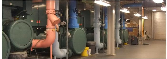
The plant provides a cooling capacity of 5,000 tons and a heating capacity of 49 MMBtu. Built with room for expansion, the CUP also houses the hospital's emergency generators and features:
