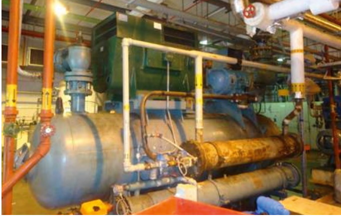
Redundant system running on R22 refrigerant
