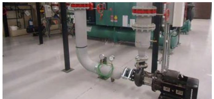
New variable-speed driven YVWA chiller unit
